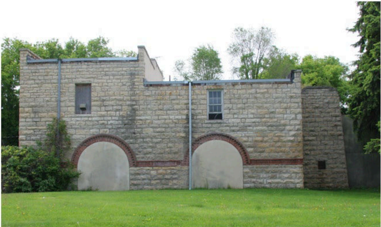
1. View to south from Levee Road
